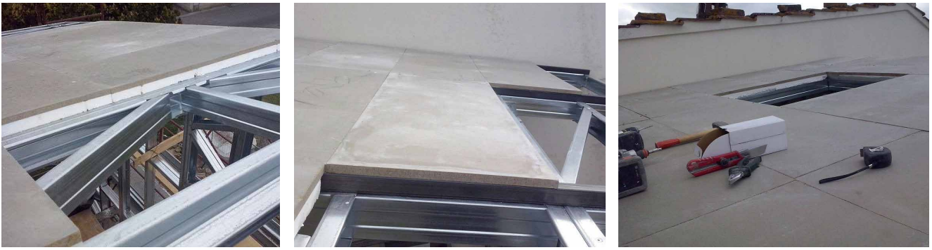
STRATIGRAPHY inverted roof with BetonStyr
